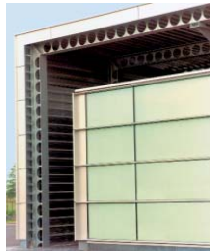
Biegesteifer Rahmen, © Arcelor Sections Cadre rigide, © Arcelor Sections
